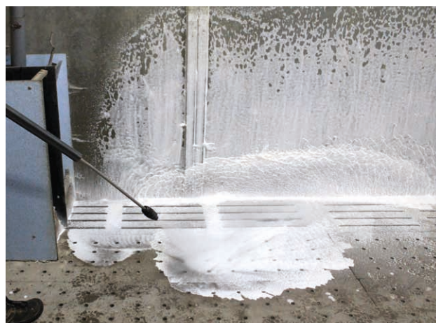
Applying Zix Eco Power with a foam unit
